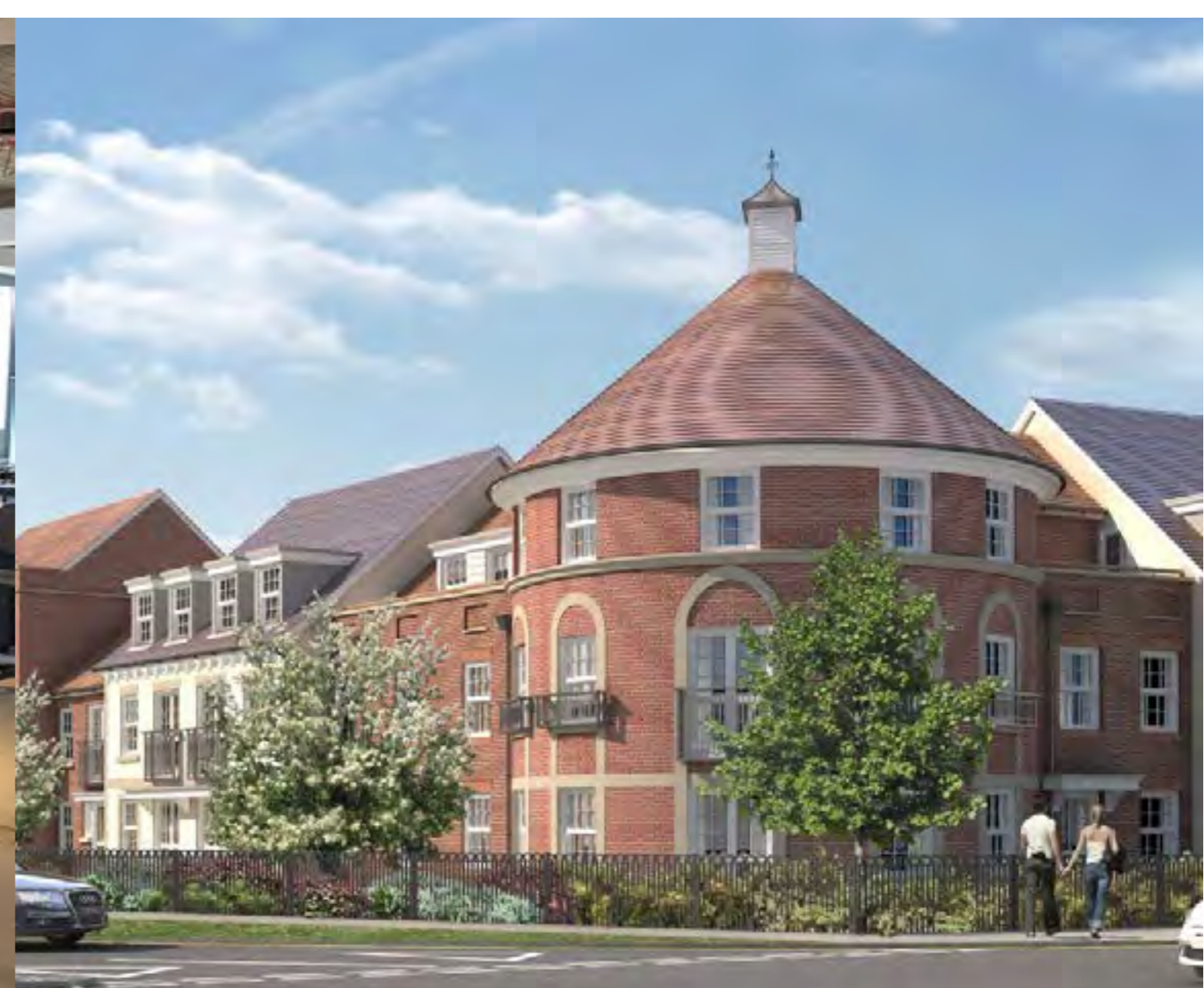
Example of a landmark building - recent housing development in Farnham
