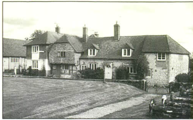
The style of windows within the group of buildings surrounding the church is generally plain casements, many with rectangular leaded lights in iron frames. Many retain original ironmongery details. Other windows are nineteenth century flush casements with horizontal glazing bars eg Roxfords House.
