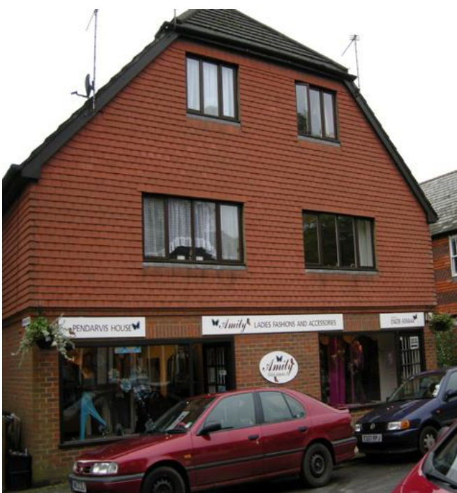
C20 building. Poor design out of character with the Conservation Area.
