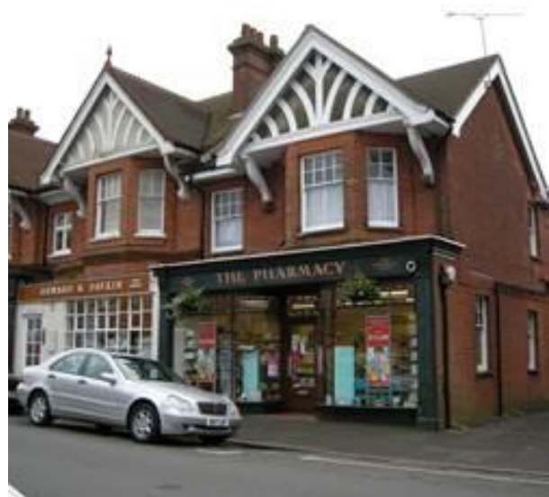
Distinctive architectural form, prominent gables, chimney stacks and a more traditional shopfront .
