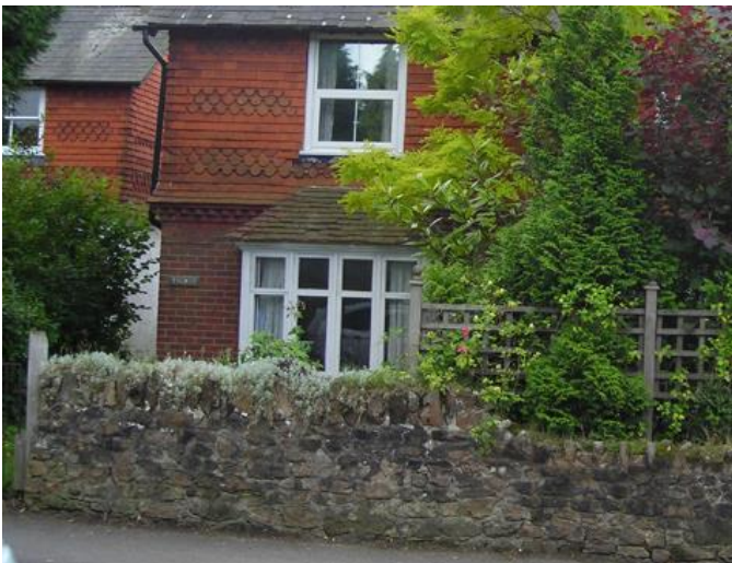
Boundary treatments - stone walls
