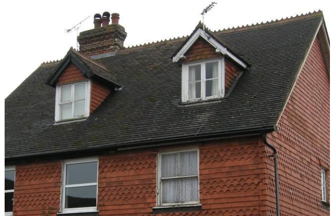
Traditional dormer windows
