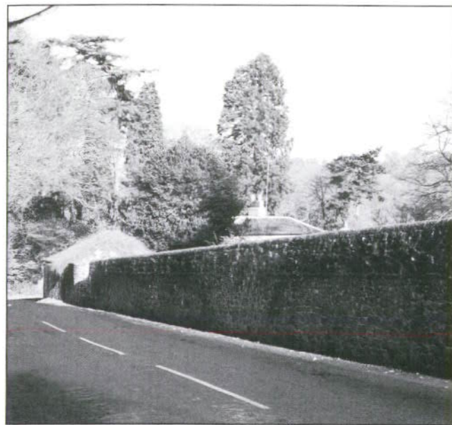
The high stone wall of Arford House is a major feature of the junction of Arford Road at Bowcott Hill where it forms a sharp bend.
