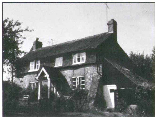
Set on the junction of Honey Lane and High Street is Pleasance Cottage , a 17th century timber framed cottage which was refaced in the 18th century. The walls are of malmstone with tile hanging on the first floor. This building is a focal point from both North and South and creates a narrow sharp bend in the road.
