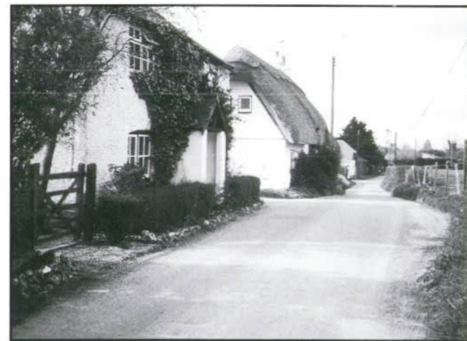
View looking north along the village street.
