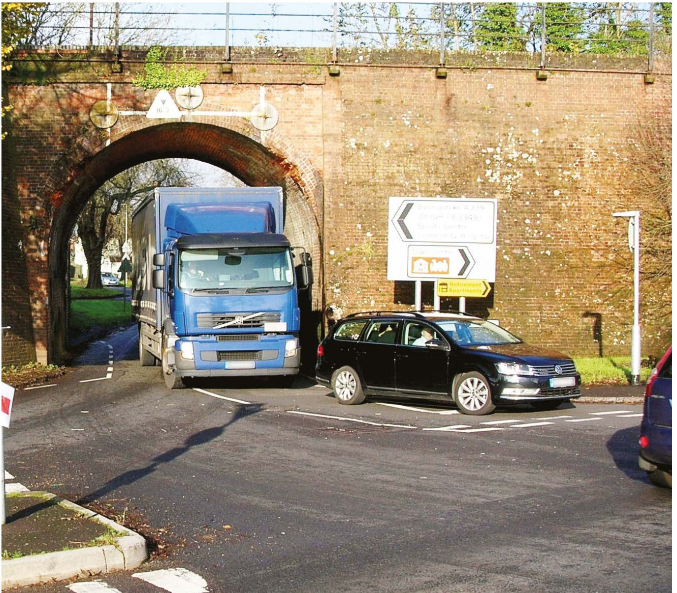
Butts Bridge – a brick arch structure.
