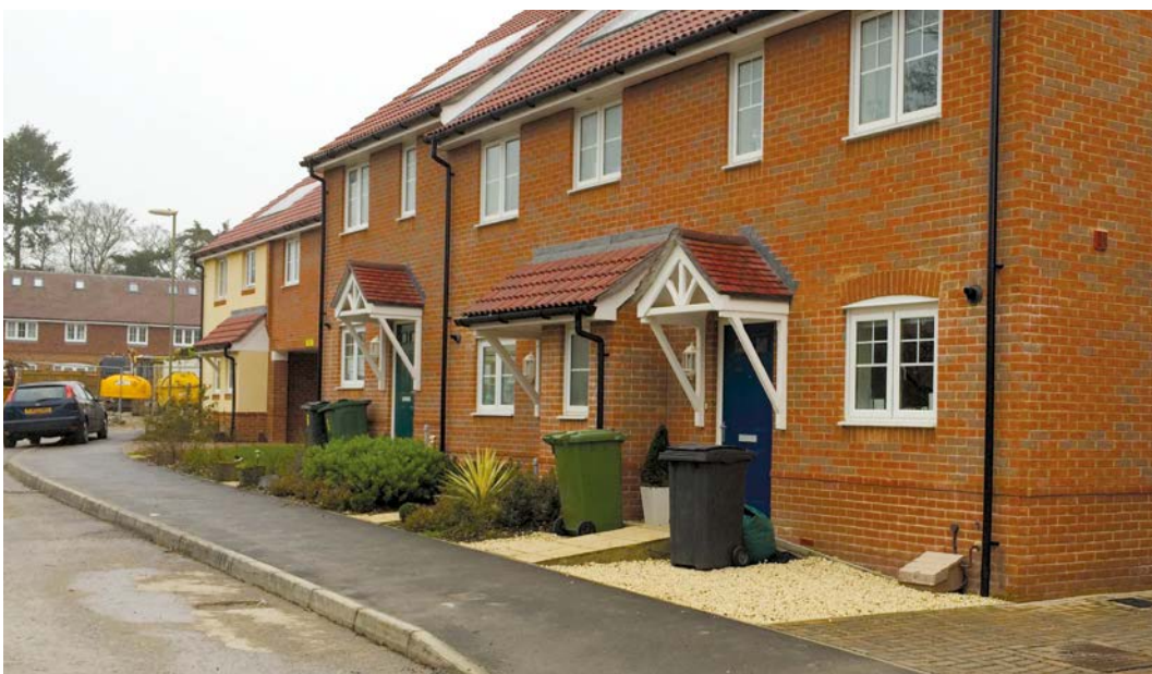
Waste Bin Storage at Barley Field Estate, Alton
