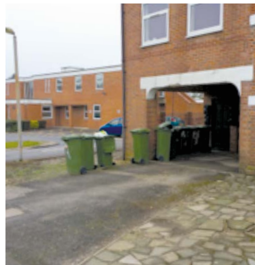
Waste Bin Storage at Anstey Road, Alton
