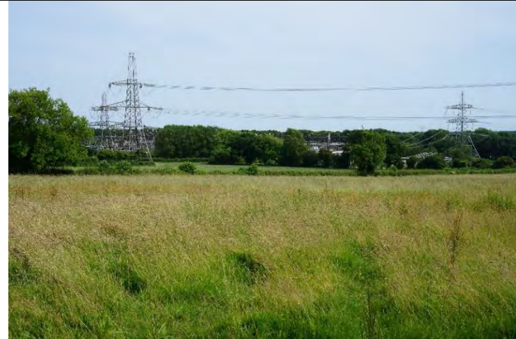
Photo 4: View looking east (from boundary of SDNP) towards substation partially enclosed by woodland
