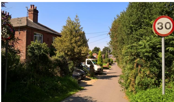
Figure 11.8 Devils Lane from the rail bridge
