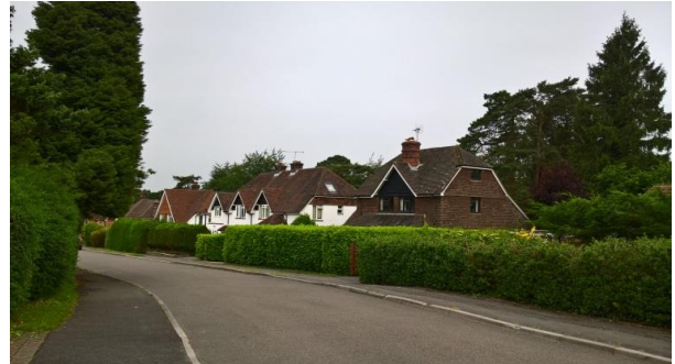
Figure 12.4 Older properties in Mowatt Road
