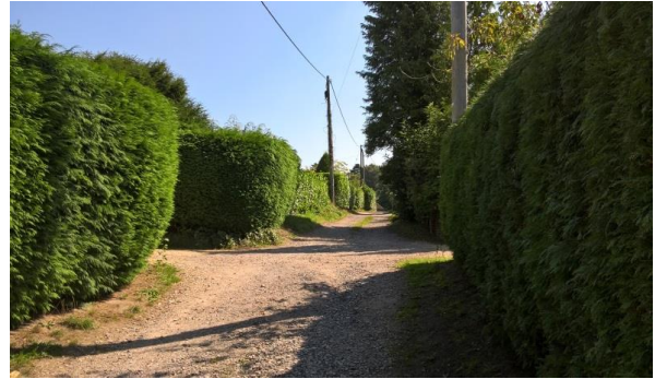
Figure 10.4 Several roads are unmade.
