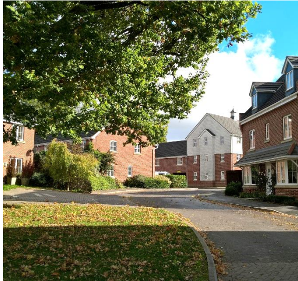
Figure 5.2 Retained open space and mature trees within housing estate - Western Four Marks
