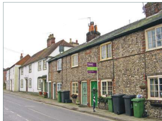
Properties on the south side of Sussex Road (Nos. 35 to 47 odd)
