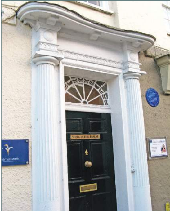
Doorcase to Worcester House, No. 2 Dragon Street
