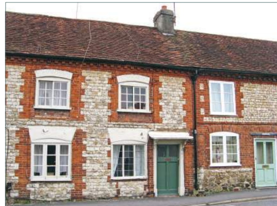
Malmstone and brick listed cottages in Sussex Road (Nos. 10 and 12)
