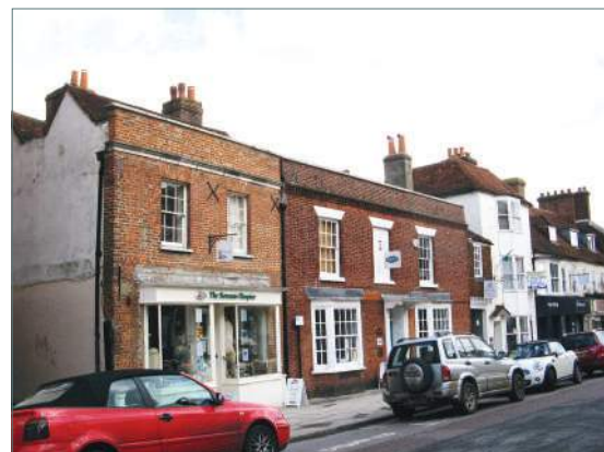
Nos. 16 and 18 High Street showing brick refronting of an earlier structure
