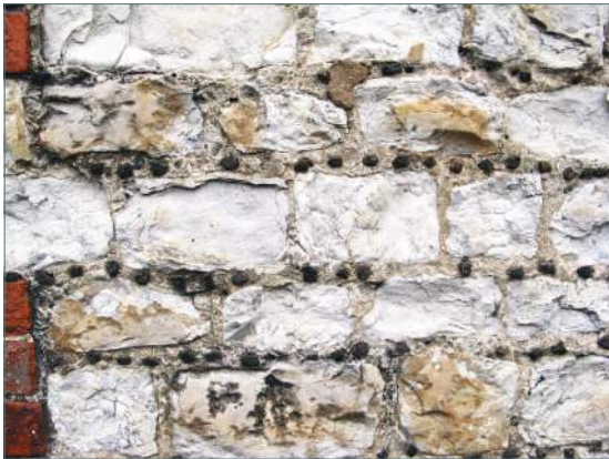
Ironstone chips used as galletting to malmstone blocks (Sussex Road)
