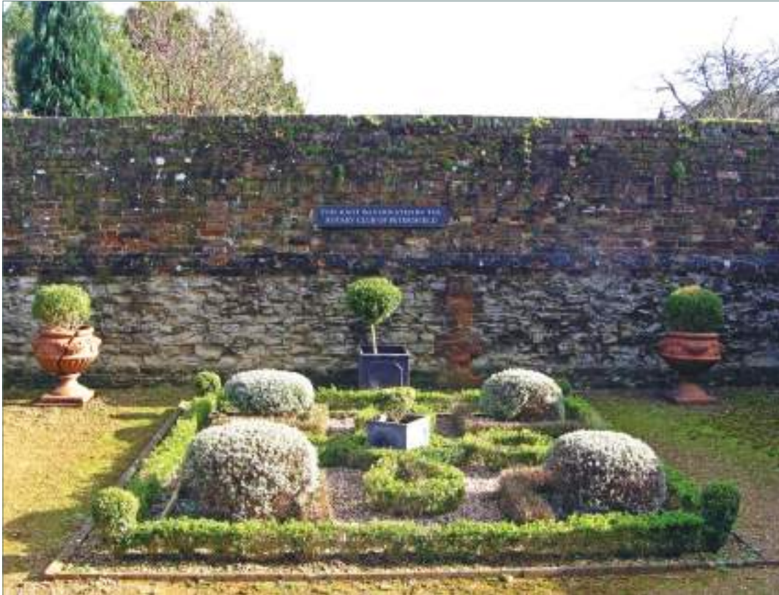
Former burgage plot wall in the Physic Garden built from malmstone and brick
