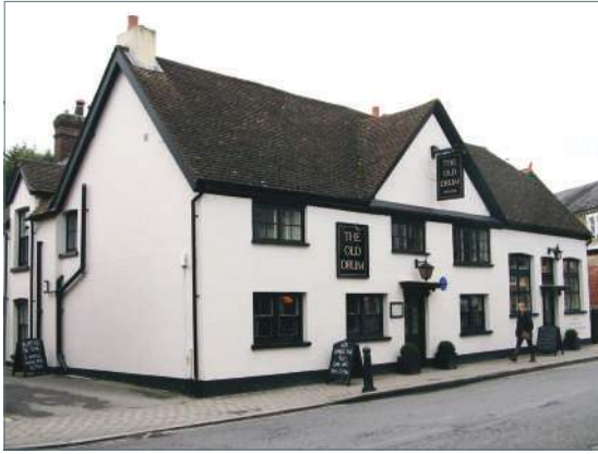
The Drum Public House, Chapel Street
