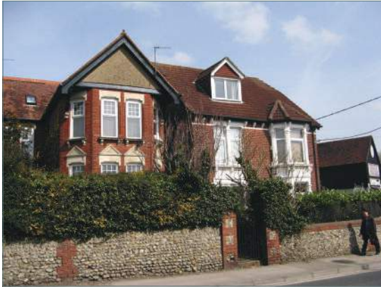
Flint boundary wall in Station Road
