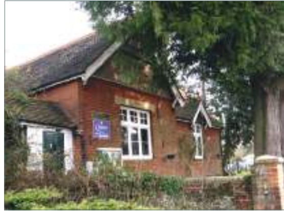
The former Men's Institute, Heath Road
