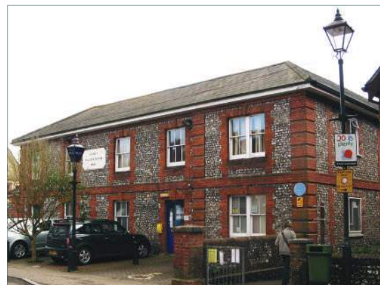
The Police Station, St Peter's Road
