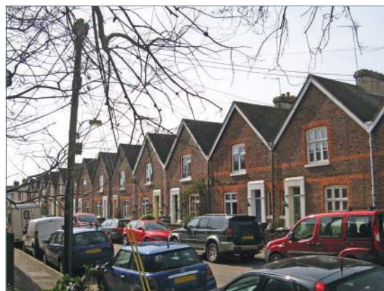
Houses in North Road
