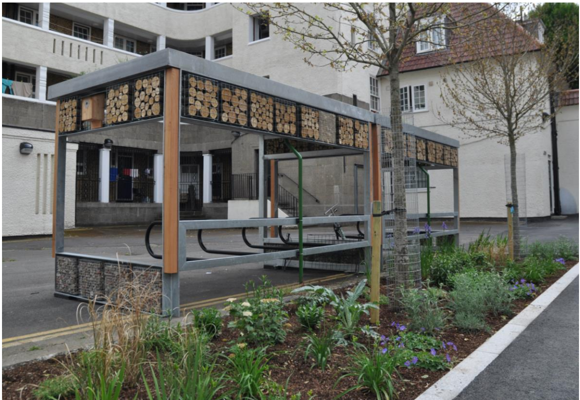
Buildings provide space for storage of bicycles and communal bins with external walls and roof used support habitats for insects.
