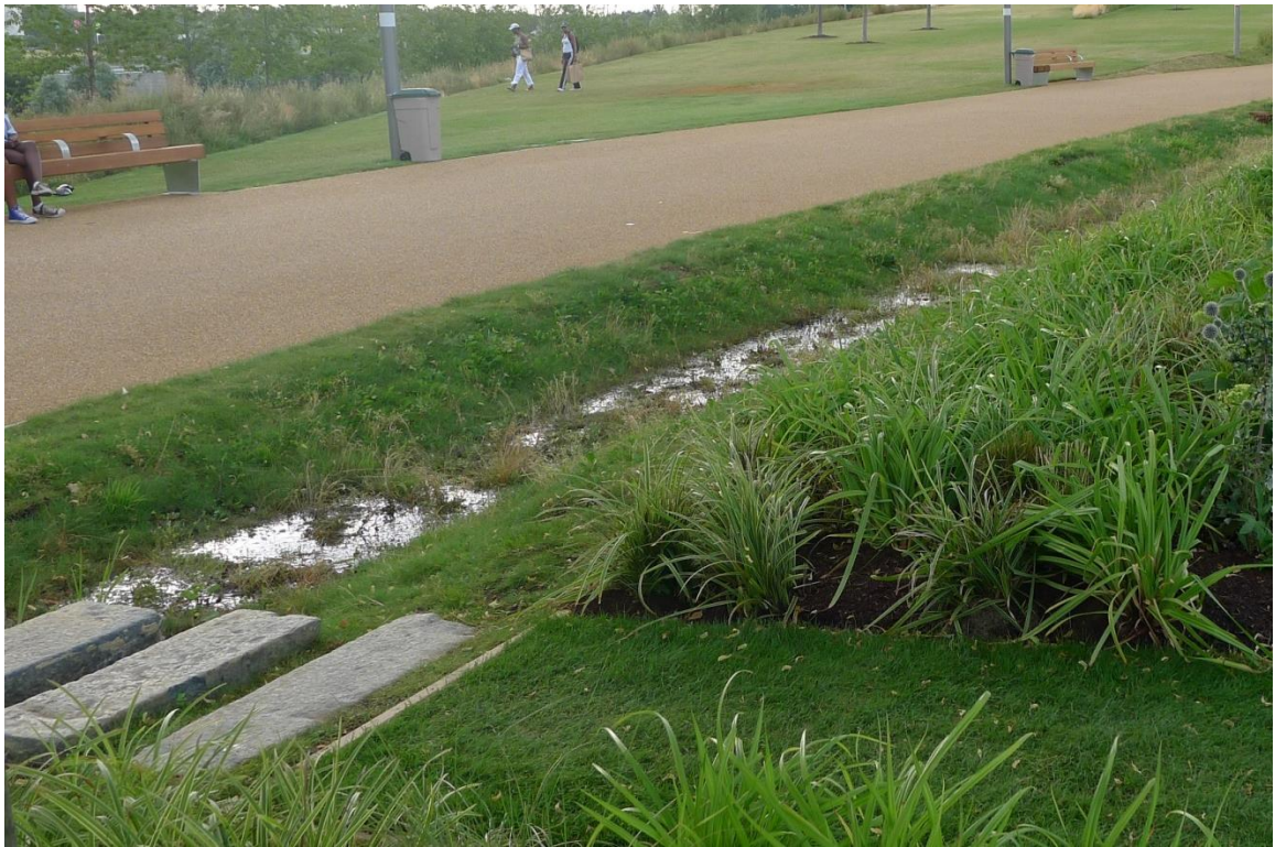
A simple swale created to one-side of a footpath to capture and attenuate rainwater runoff.
