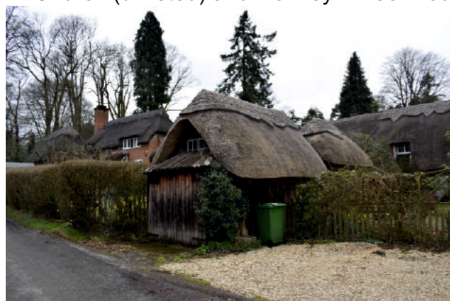
Listed buildings on Wellhouse Road
