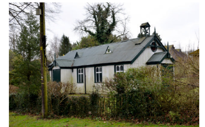
St Peter's Church dating from 1902 one of few remaining pre-fabricated buildings within the village
