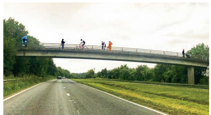
Utilising existing A31 bridge crossing to link Neatham Down to Alton
