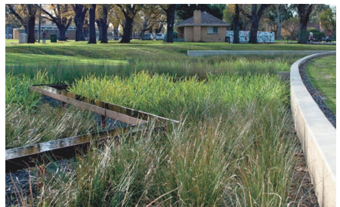
Examples of Sustainable Urban Drainage Systems (SuDs) such as bio swales and rain gardens.
