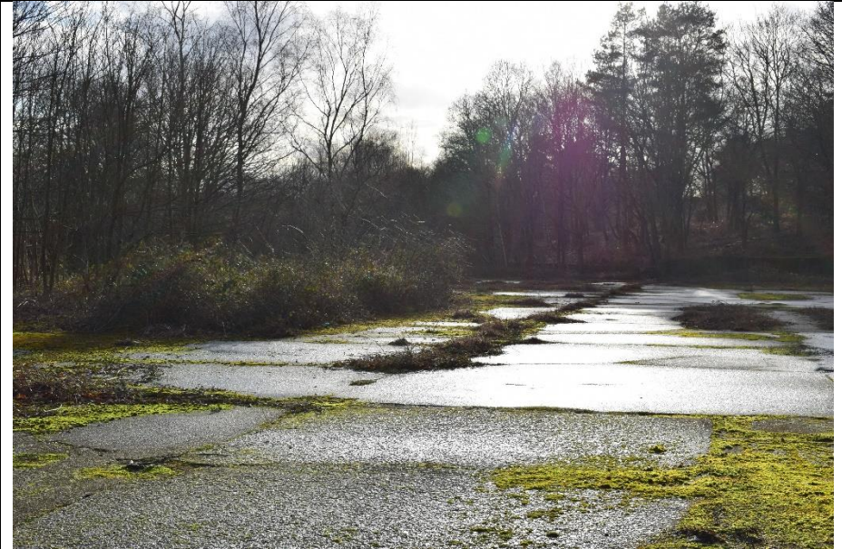
Photo 6: View south-west from Broxhead Farm Road across hardstanding towards Oakhanger Road towards Broxhead Common South and West SINC.
