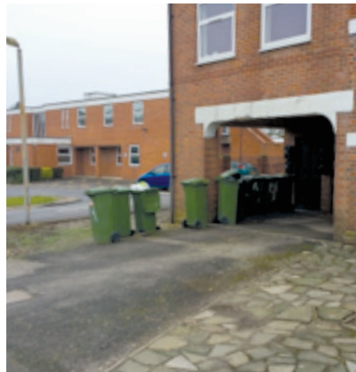
Waste Bin Storage at Anstey Road, Alton
