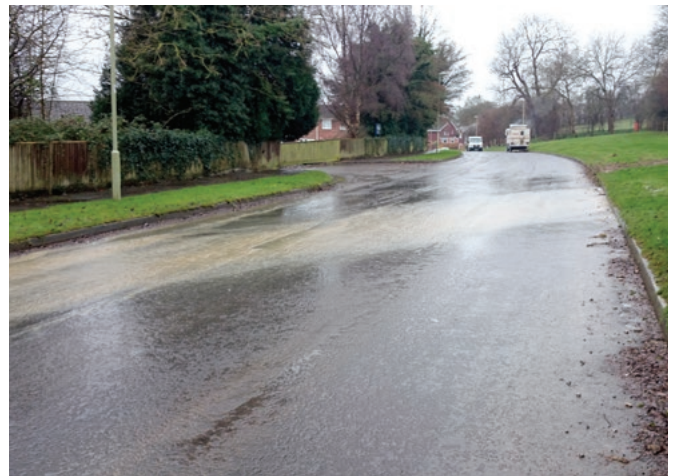
Evidence of rain water run-off leading to flooding from high ground in North Alton across Gilbert White Way
