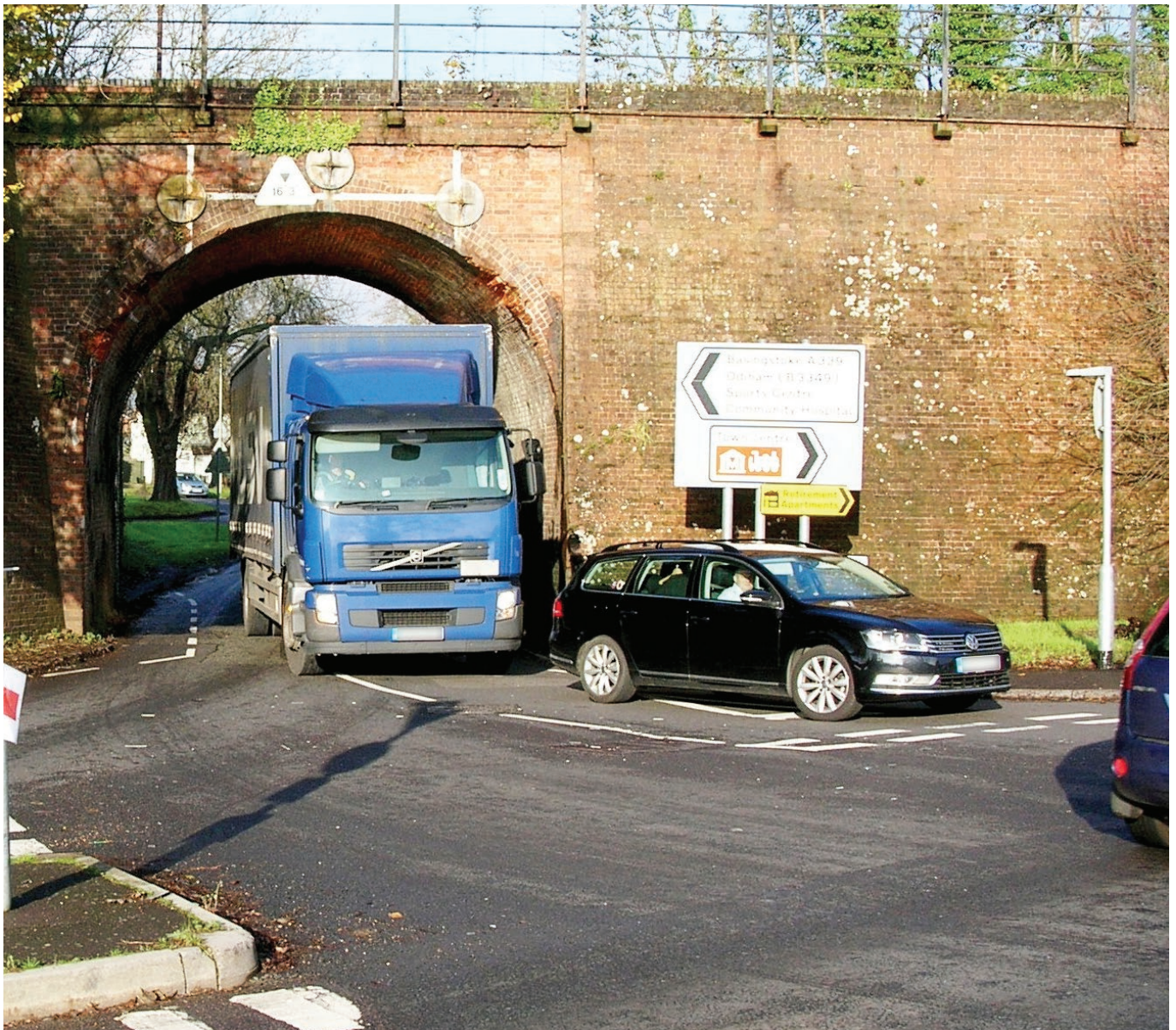
Butts Bridge - a brick arch structure.
