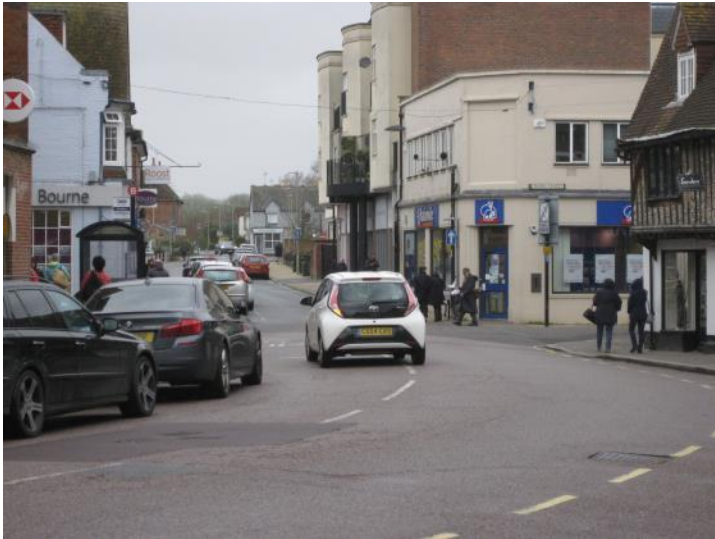
Figure 9: The junction of the High Street, Swan Street and Chapel Street looking west. The parked cars (and sometimes buses) force westbound drivers into the opposite carriage thus creating a collision risk. (This photograph was taken in 2019).
