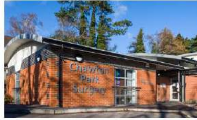
Local GP Practice in Alton allocated CIL funding in 2022 (Photo provided by Studio Four Architects)
