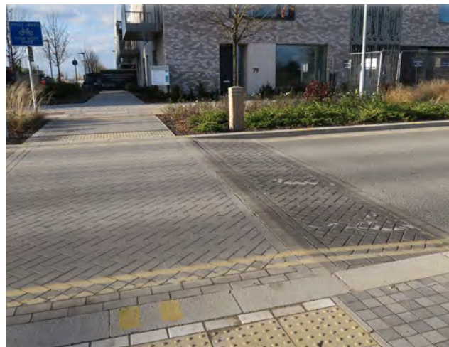
Figure 39: Example of a raised pedestrian crossing on a main road, with contrast paving materials and space for low-level planting and with contrasting paving materials.
