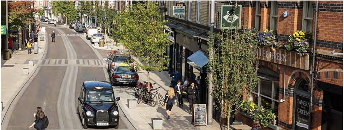
Figure 42: Stamford New Road after reconstruction in Altrincham. The new design re-organised traffic flows by introducing a central median, installing new trees and planters, adding crossings, using high-quality paving materials, and rationalising car parking (Source: https://www.bing.com/images ).
