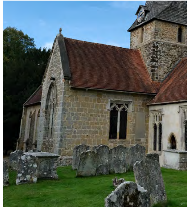
Figure 12: St Mary's Church in Bramshott with stone walling.
