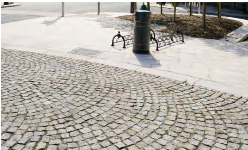
Figure 43: Paving transitions between main pathway and furniture zones.
