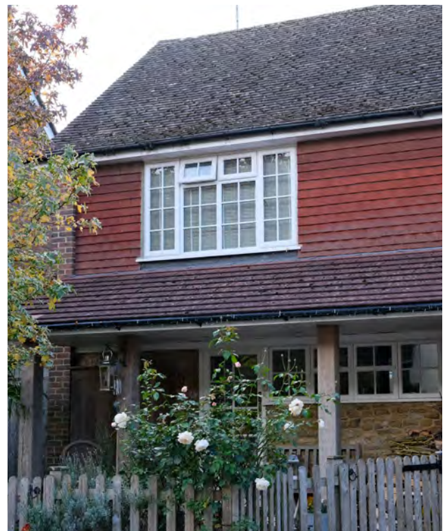
Figure 13: Property in Bramshott which has typical hung tiles on the building facade.
