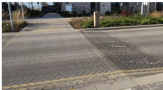
Figure 62: Example of a raised pedestrian crossing on a main road, with contrast paving materials and space for low-level planting and with contrasting paving materials.
