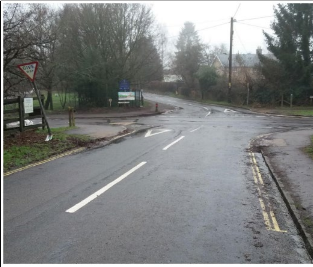
Figure 7.1: Alton Lane, Five Lanes area of Four Marks
