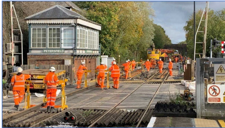
Figure 6: Engineers working on the S&C renewal near Petersfield station (Network Rail)
