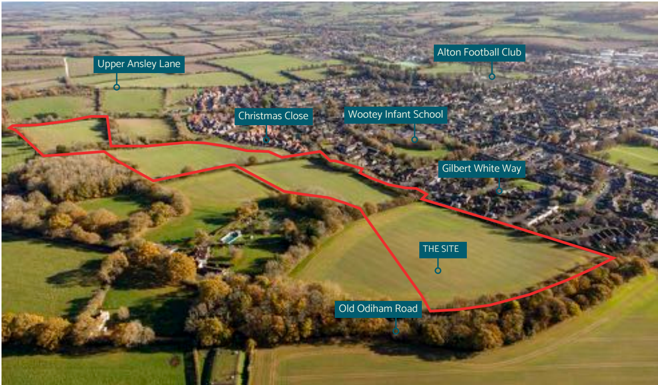
View looking south-east across the site
