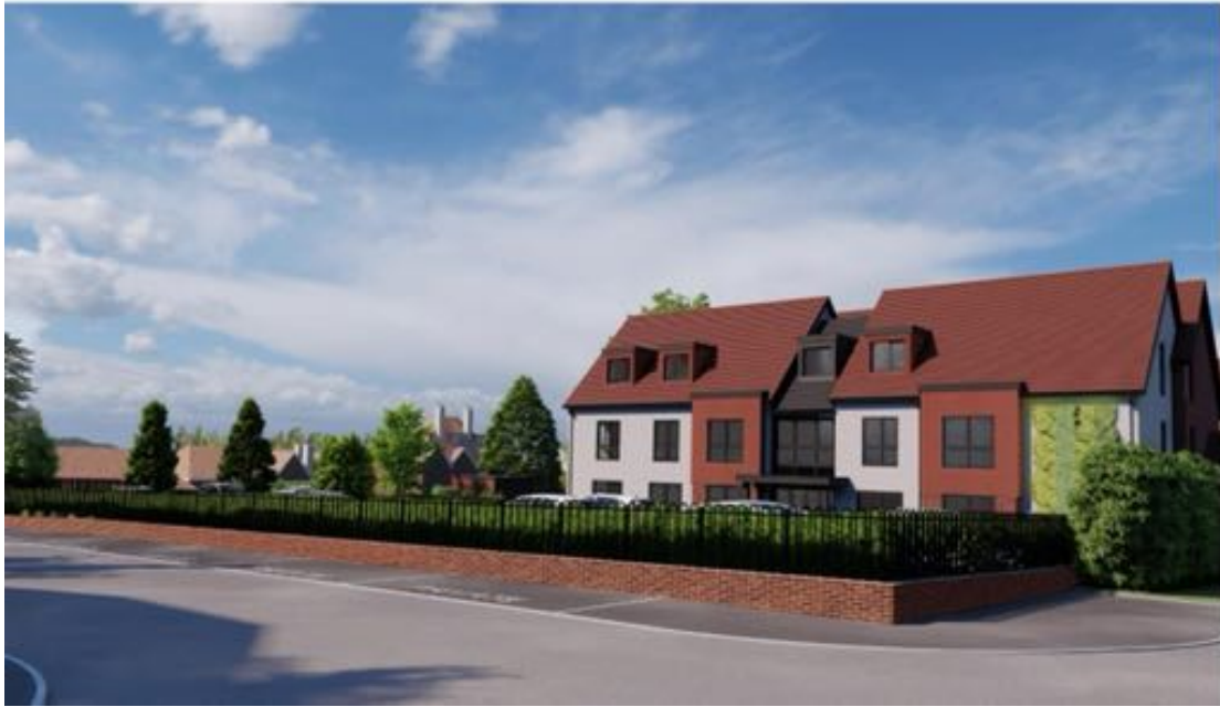
Extract from 3D Visual showing view of the refused care home from Royal Huts Avenue
