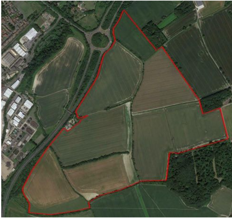
Figure 2.2. Aerial imagery of the site.
