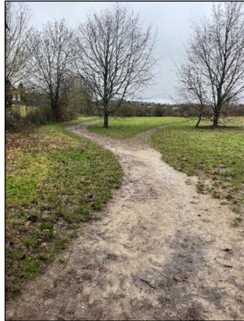
Photograph 20: Existing conditions of Sunderton Lane Meadow footway
