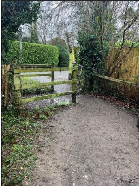
Photograph 19: Existing conditions at Sunderton Lane footway access
