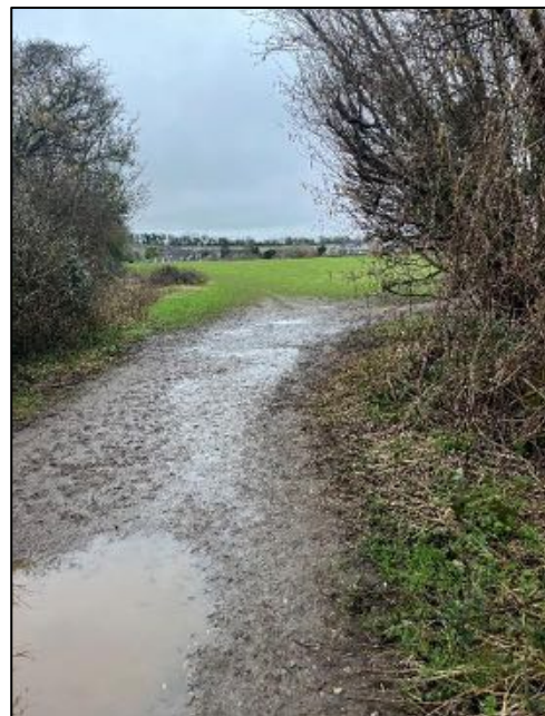
Photograph 22: Existing conditions of South Lane Meadow footway
