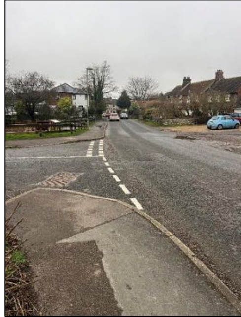
Photograph 10: Queuing along Chalton Lane at 15:30pm
