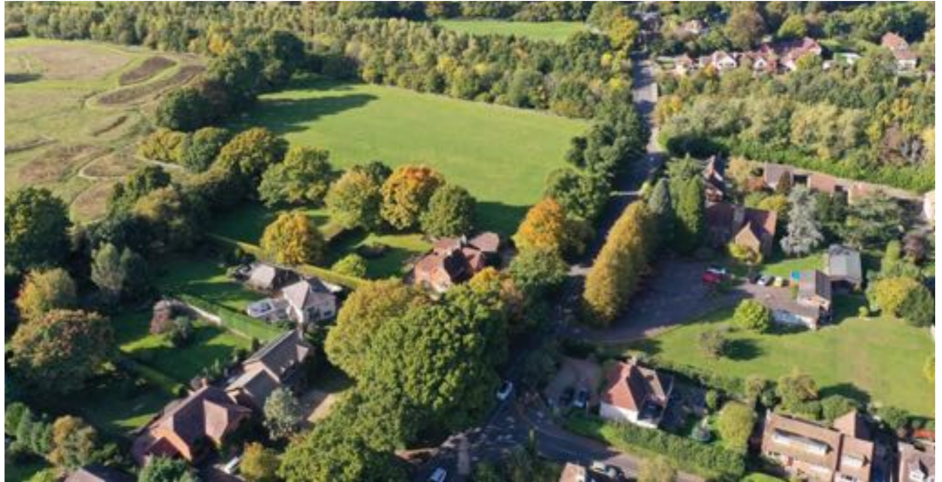
1. Aerial view of the Site looking north west
