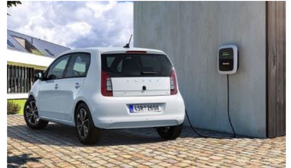
EV charging points through out the site
