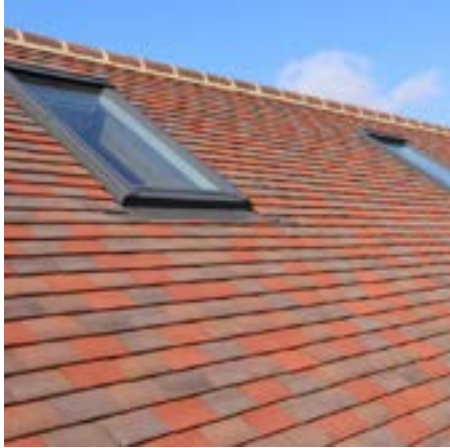
Red/brown roof tiles
