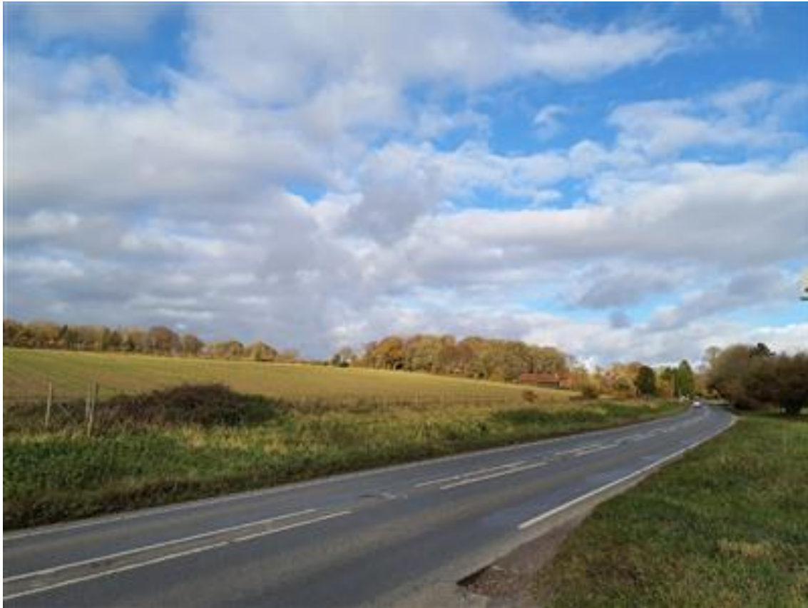
Figure 5.9: Large undulating arable fields adjacent to the A31 north of Ropley enclosed by trees and woodland
