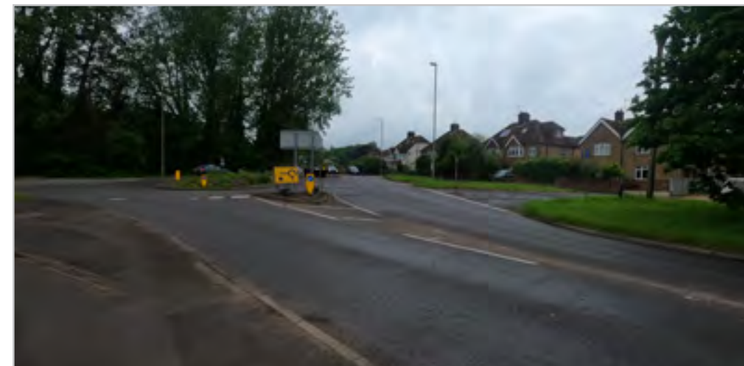
WR3.3.13 – Winchester Road leading up to the roundabout
