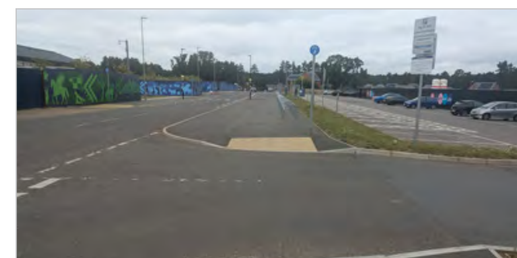
Example 2 – Straight alignment of Havannah Way, consider speed environment and continuous footways
