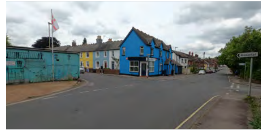
WR3.9.17 – Junction of Swan Street and Charles Street
