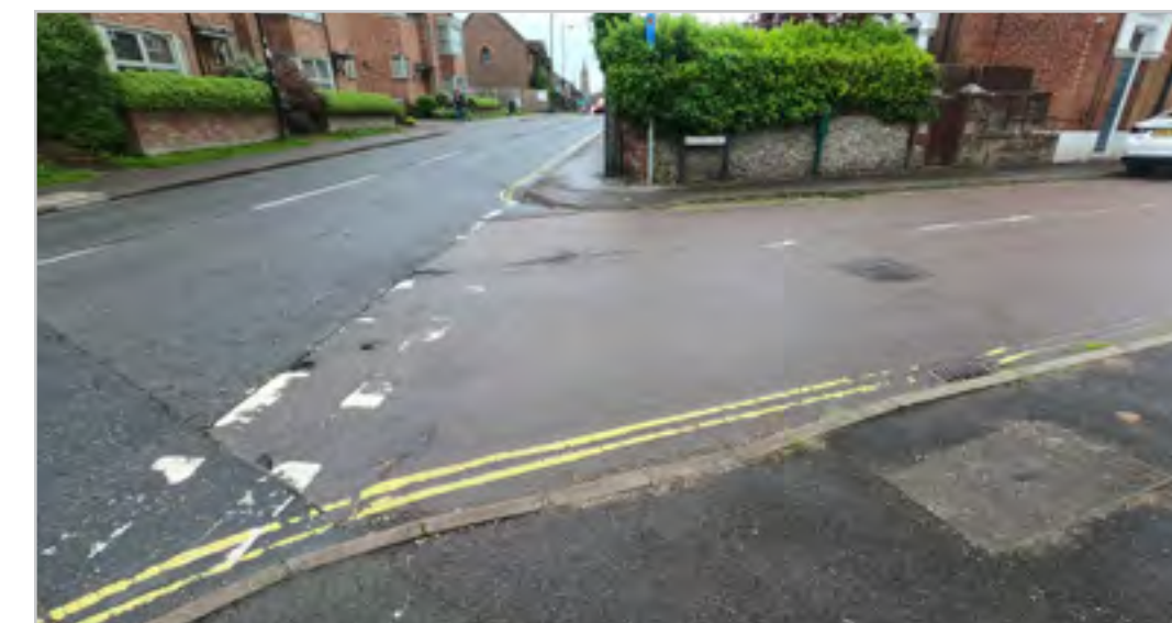
WR3.4.9 – North Road and Station Road
