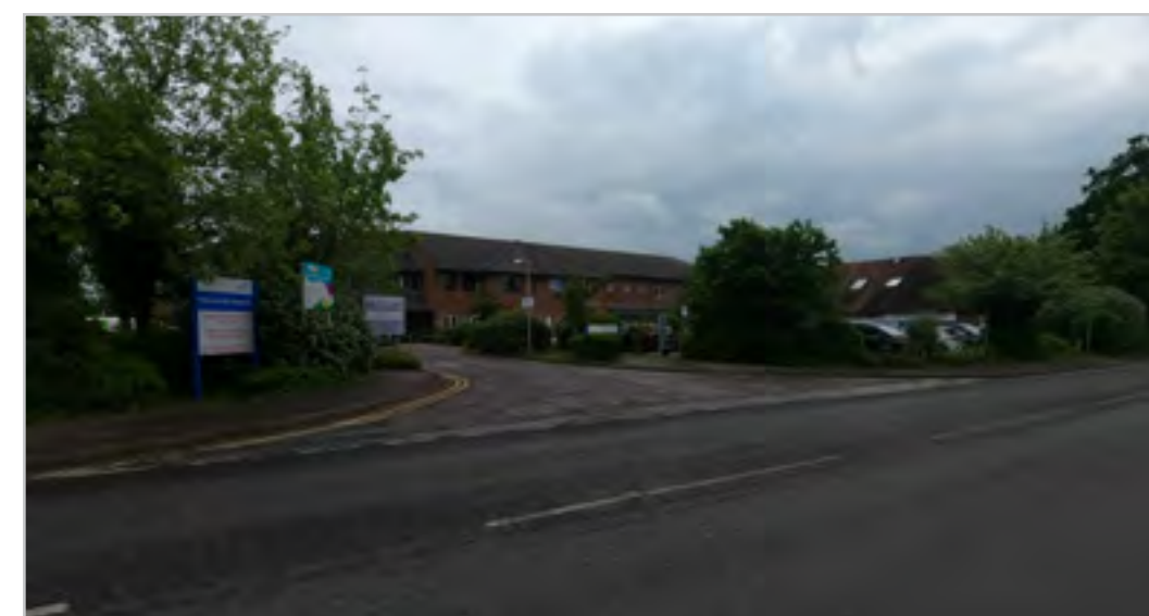
WR3.2.4 – outside Petersfield Hospital
