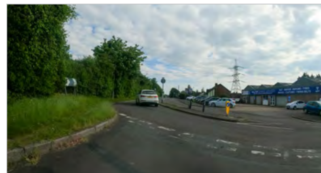
110.6.5 – London Road / Drift Road junction
