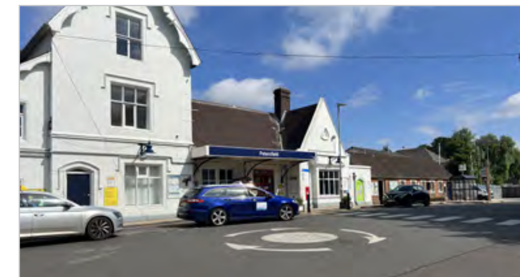
WR3.3.7 – Petersfield railway station
