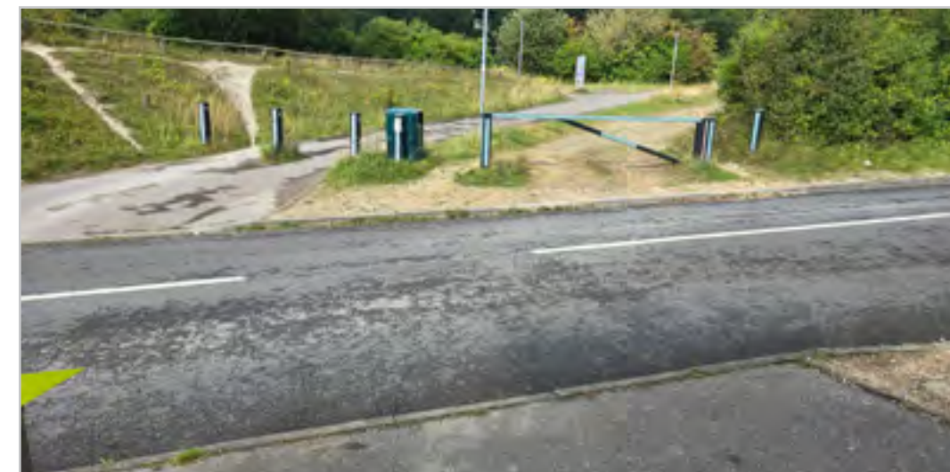
110.5.8 – South Downs Way off road access junction
