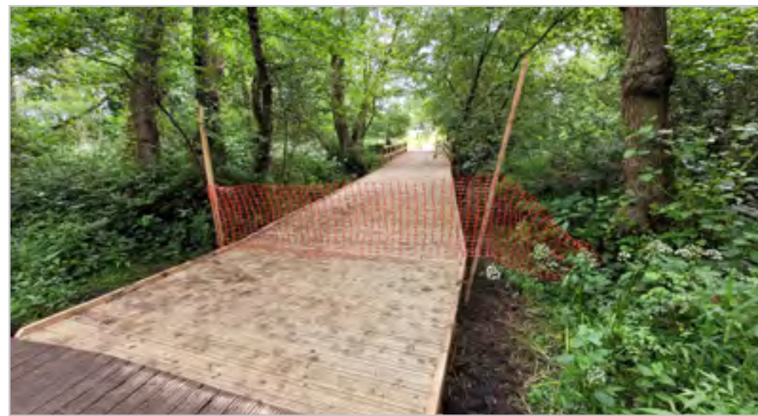
WR2.1.6 – Lindford Link Bridge
