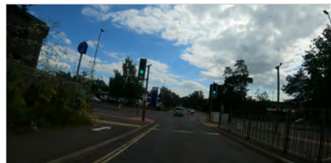
100.1.8 – High Street recently widened shared use path
