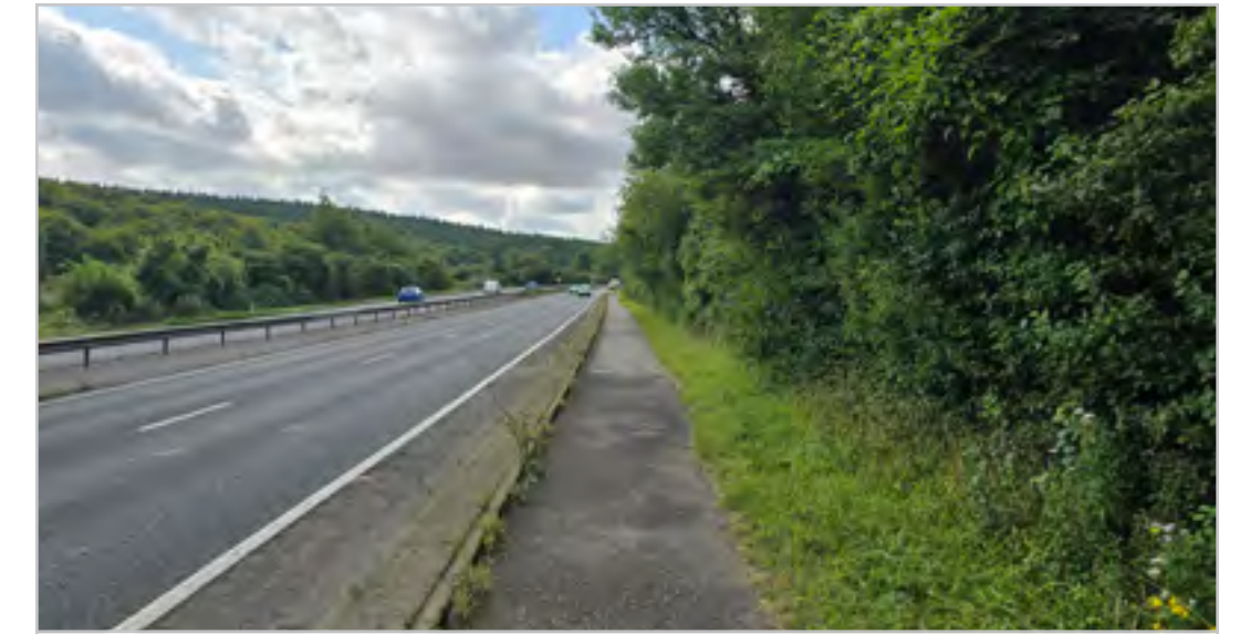
110.5.10 – A3 junction to Gravel Hill
