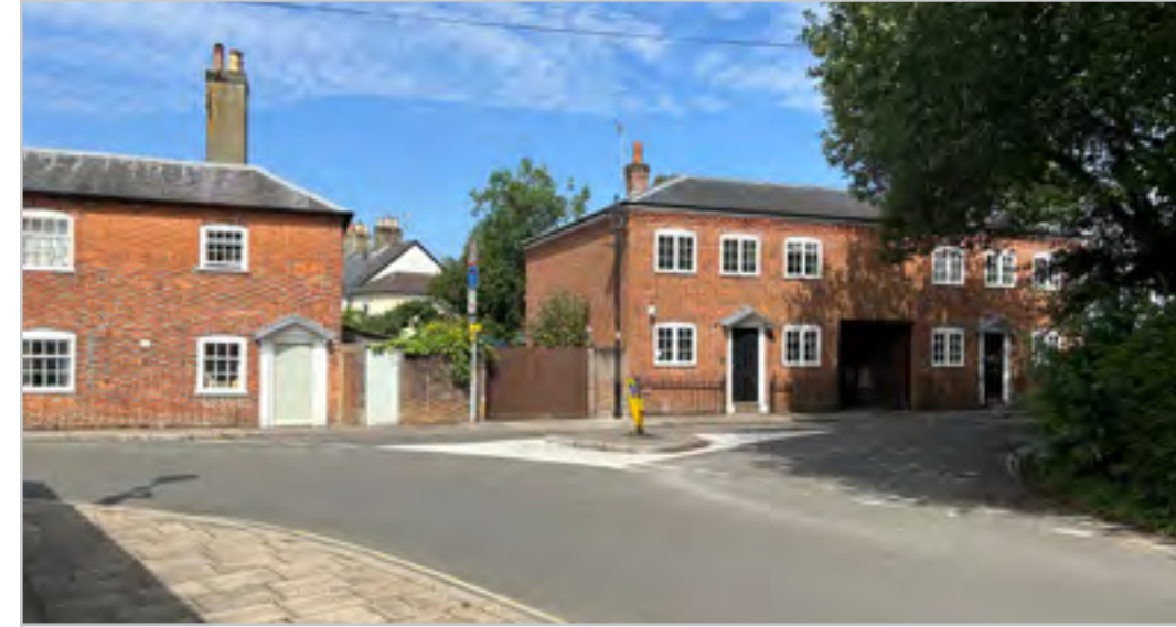
WR1.6.15 – Amery Hill/Amery Street junction
