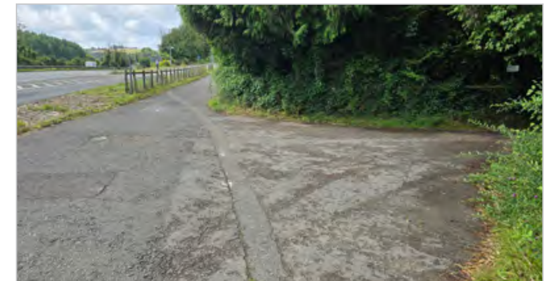
110.5.11 – A3 junction access path to Gravel Hill
