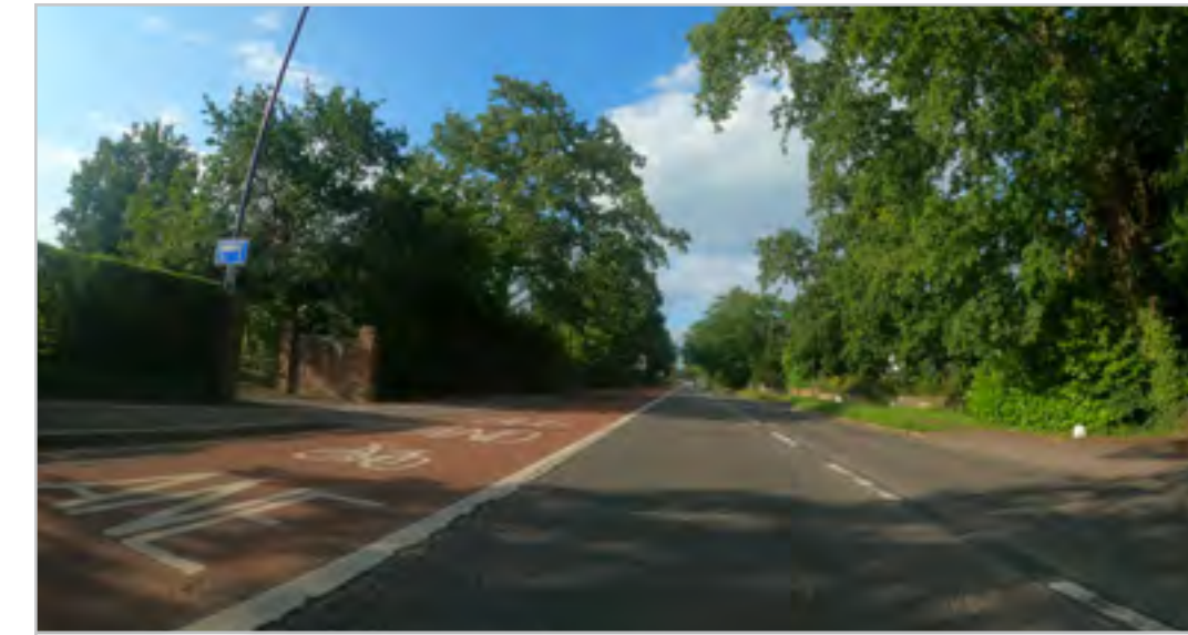
120.1.6 – Portsmouth Road (A3)
