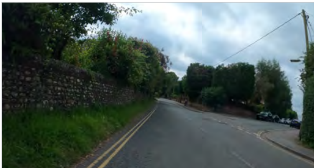
220.3.3 – Heath Road / The Courtyard
