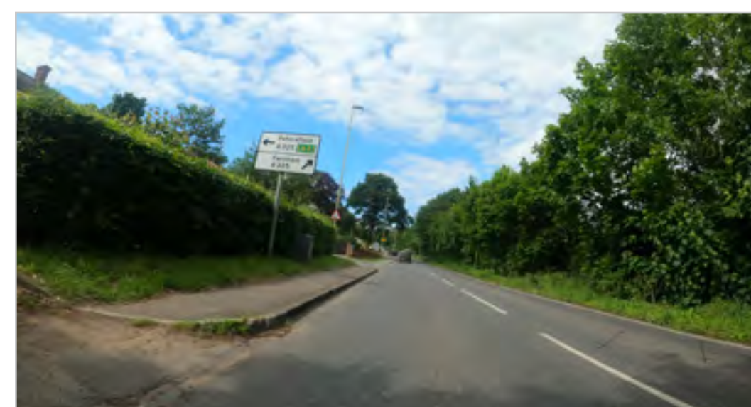
110.1.2 – B3002 Farnham Road pavement
