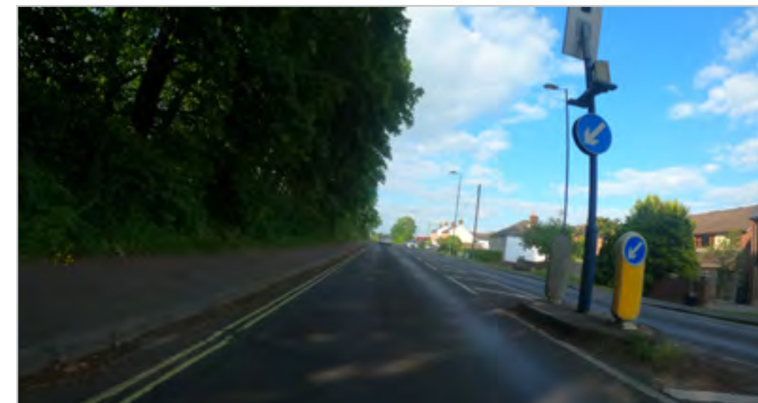
120.1.4 – Portsmouth Road (A3)
