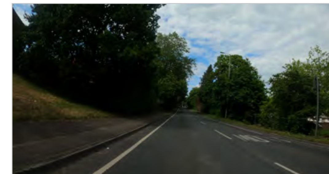
100.1.4 – Camp Road pavement
