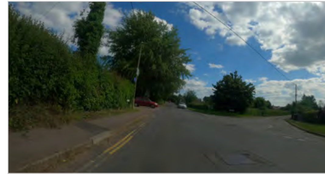
110.2.12 – Hill Brow Road/Andlers Ash junction
