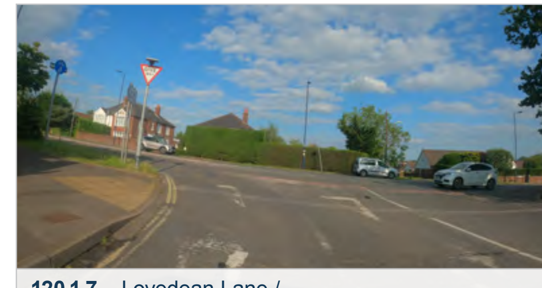
120.1.7 – Lovedean Lane / Prochurch Road junction
