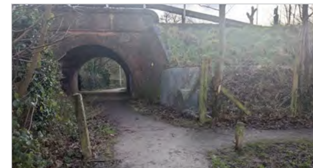
110.3.16a – Railway underpass
