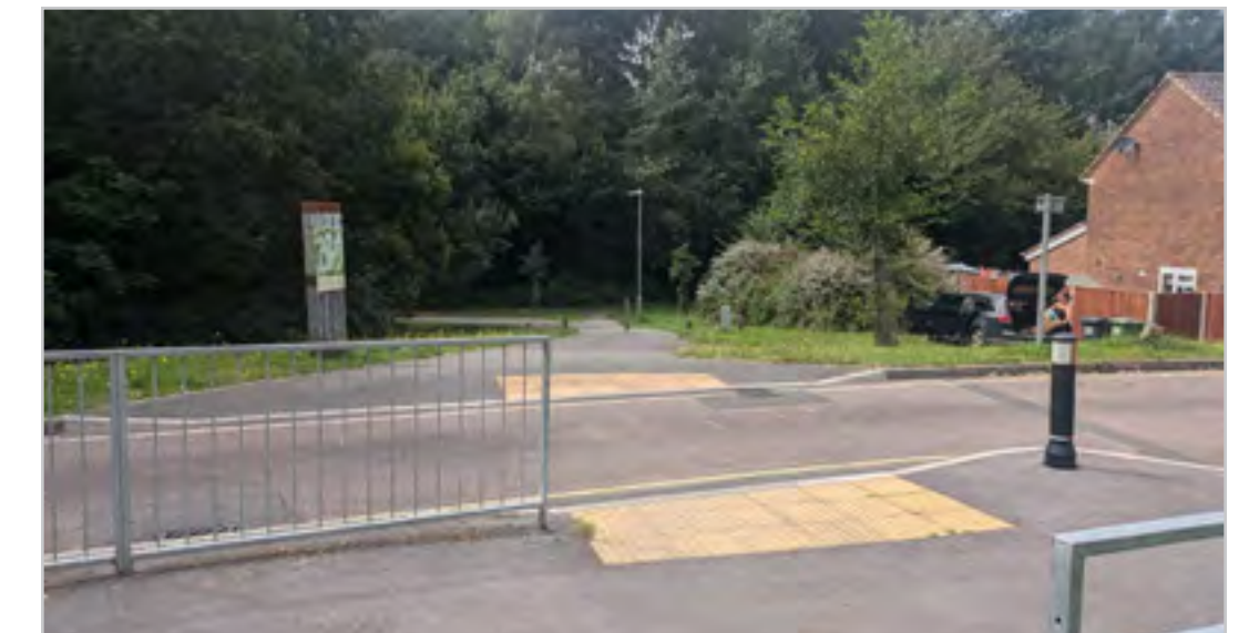
WR2.4.9b – Oakley Road uncontrolled crossing
