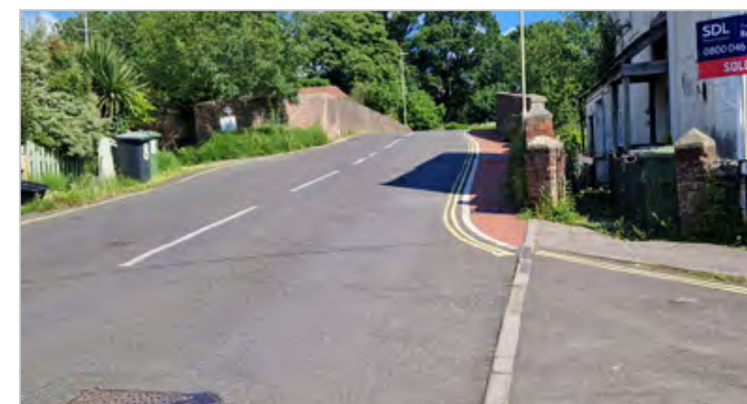
110.4.4 – Tilmore Road railway bridge
