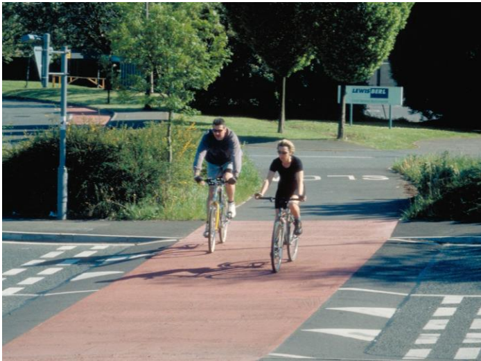
Priority cycle path crossing of minor road (Photo: J. Bayne/Sustrans www.sustrans.org.uk )
