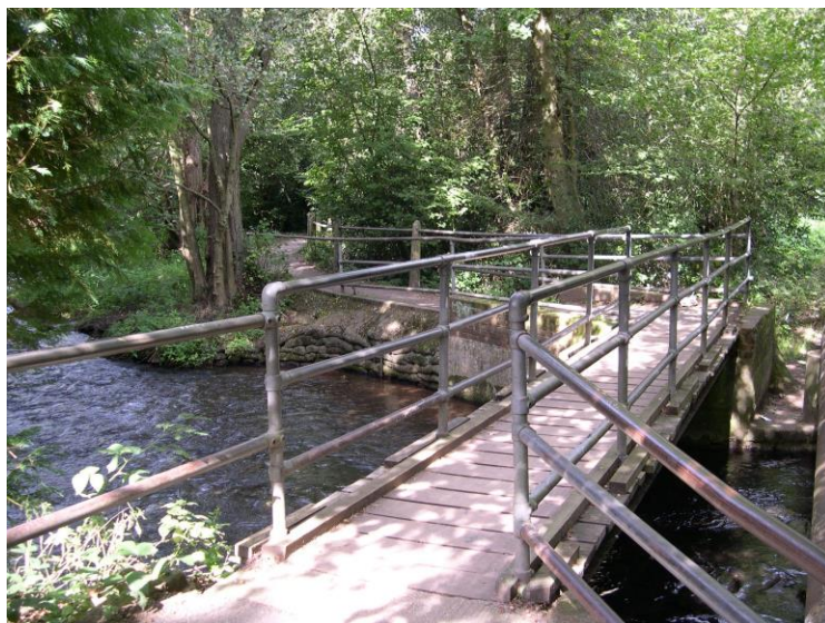
Washford Lane footbridge
