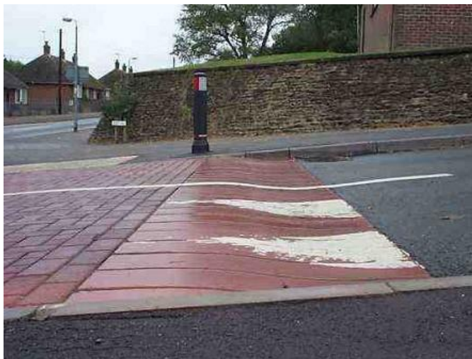
Sinusoidal road hump. (Photo: D. Kemp/Sustrans www.sustrans.org.uk )
