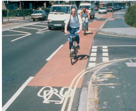
Cycle lane continuity across a junction Portsmouth, Hampshire (Photo: Sustrans www.sustrans.org.uk )
